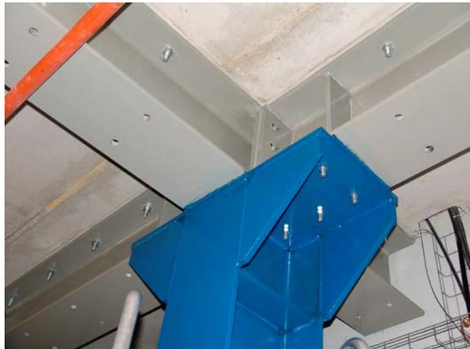
Figure 9. Example of link between columns, beams and concrete slab.
